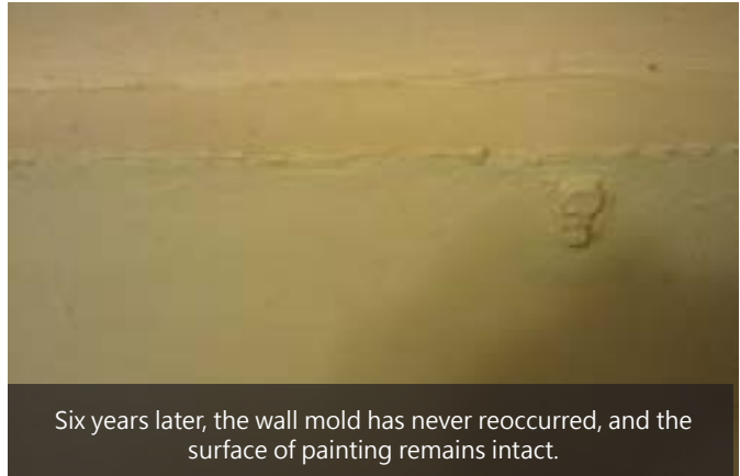
This is an indoor construction project for the purpose of preventing wall mold due to moisture in the mountains.
