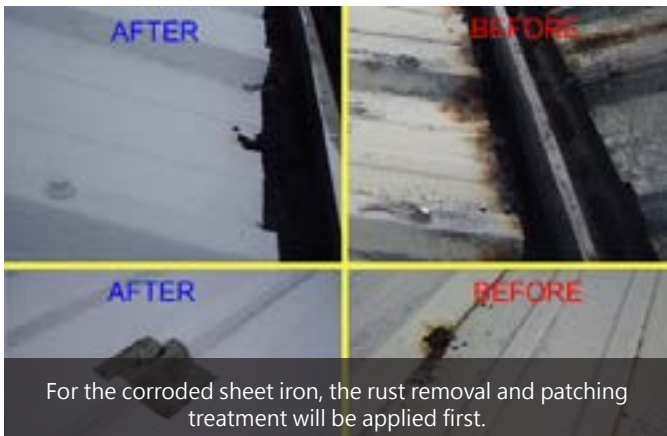
The HeatAX nano heat insulation coating can provide the protection against worsening corrosion and prolong the service life of building.
